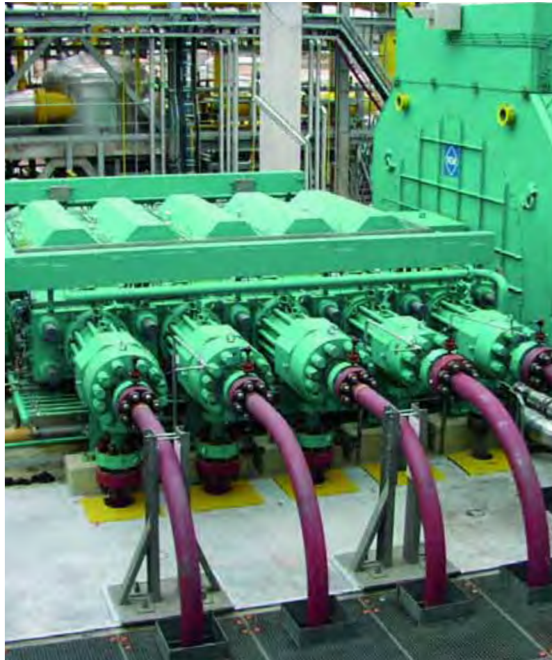
The RotaBolt design can dramatically speed up routine maintenance checking on this hyper compressor from Burckhardt Compression
