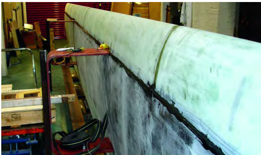
Bonding of sail's U-shaped leading edge assembly to central box
